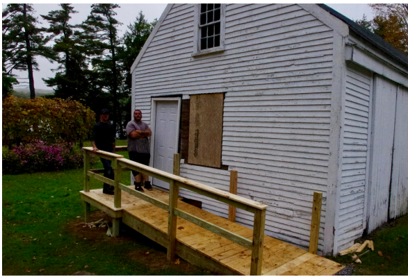
The newly remodeled Carriage House bathroom will be wheelchair-accessible.
