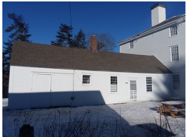
The Court House Ell sports a new roof.
